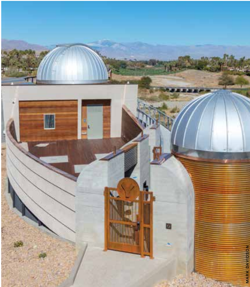
Above: The design of the Observatory incorporated materials to create a beautiful and durable structure that will hold up to the desert climate. The exterior of the Observatory structure is clad with stucco, corten steel, and copper cap flashings. The viewing deck and walls are covered with a very dense hardwood: Brazilian IPE. The structure is built with concrete caissons, concrete walls, steel post and I-beams, and heavy gauge steel studs. Right: The Rancho Mirage Observatory houses the PlaneWave CDK700 telescope, a revolutionary optical system with innovative technology of the highest quality.
